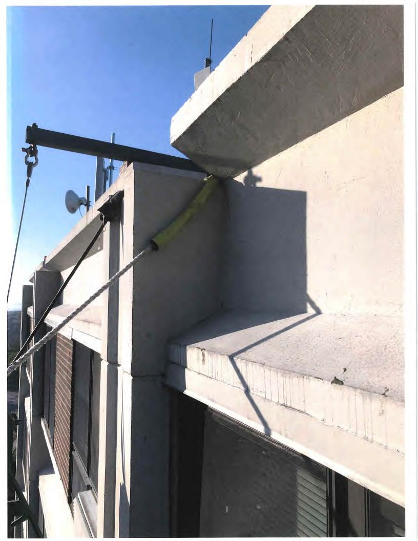
TOP OF CONCRETE COLUMN DETERIORATION NEEDING REPAIRED
