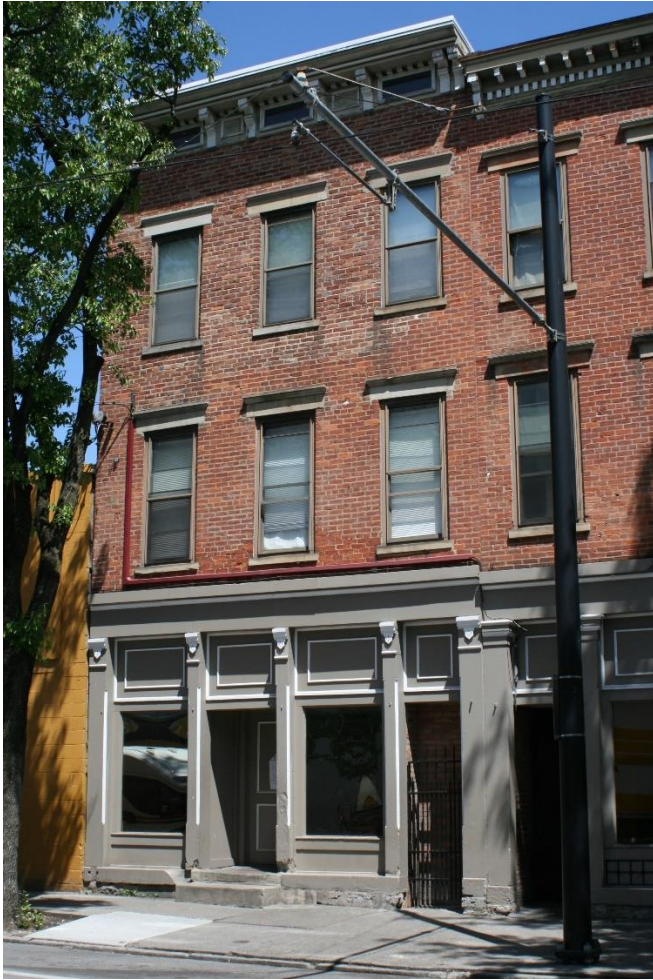
West Façade – North Side
