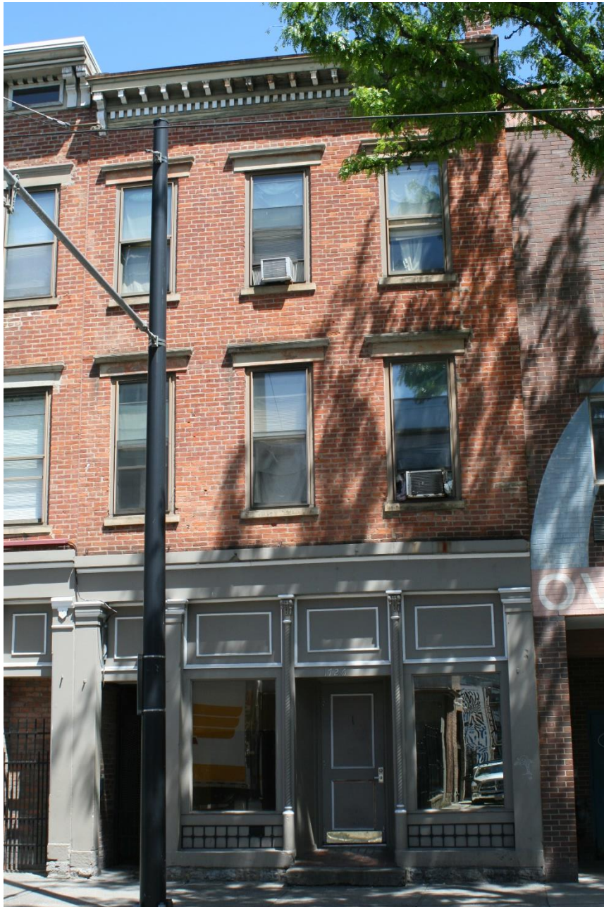
North Façade – South End
