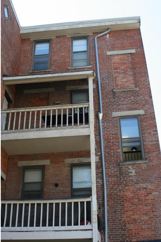
East Façade – North Side
