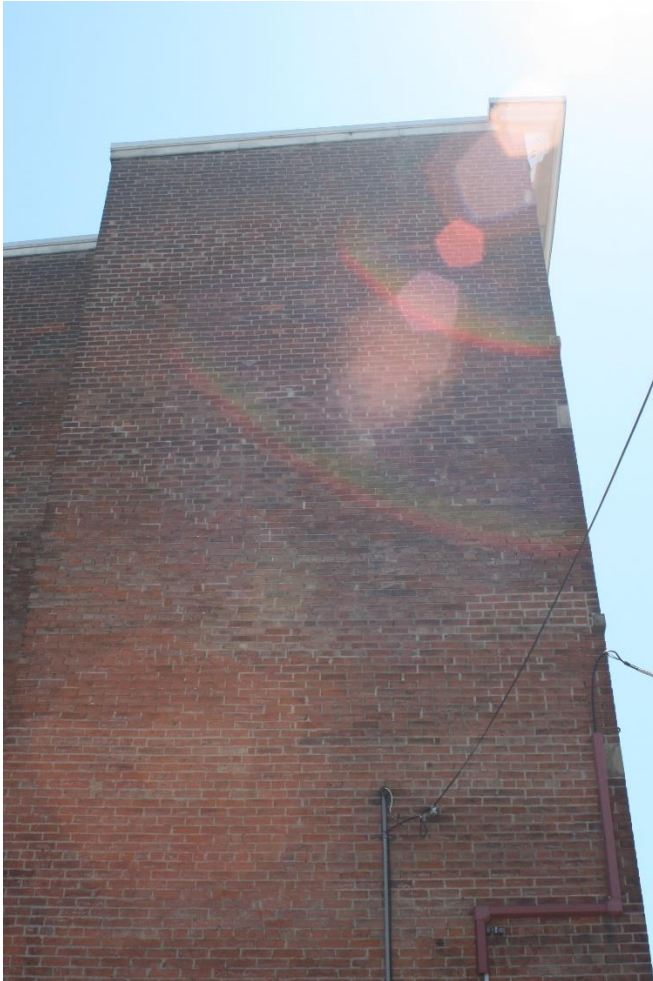
North Façade – Race Street Side
