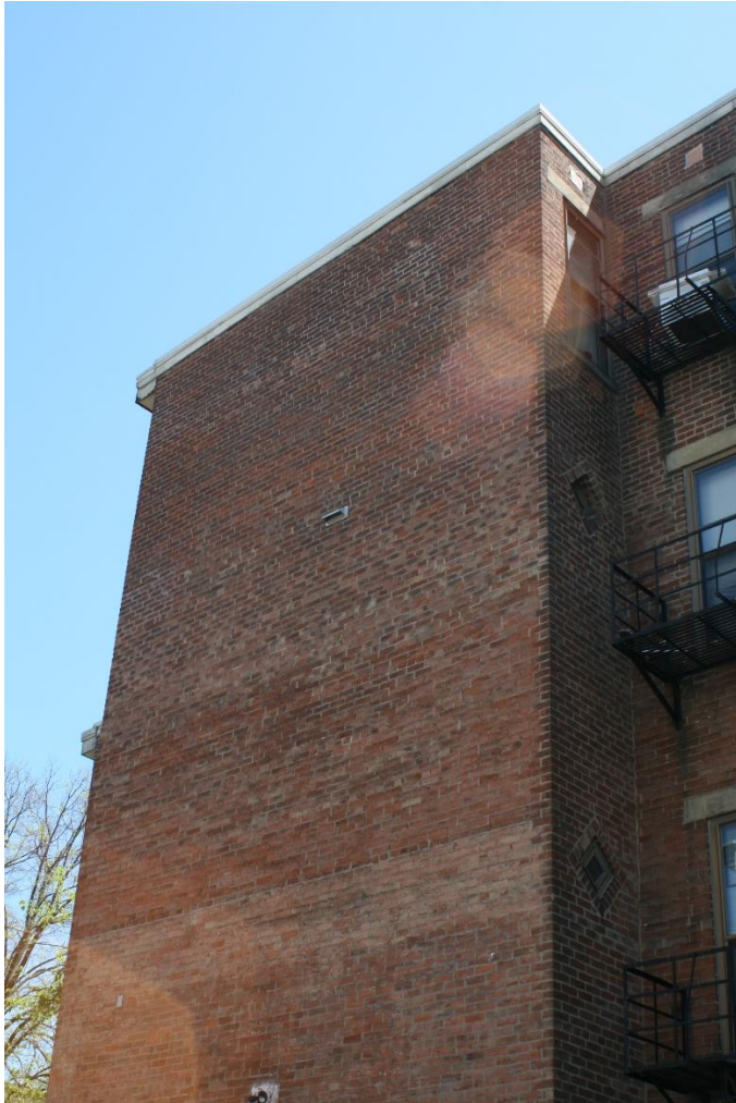
North Façade – Goose Alley Side
