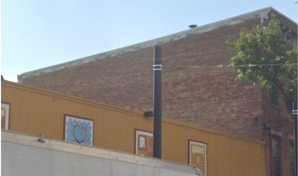
North Façade – Race Street Side
