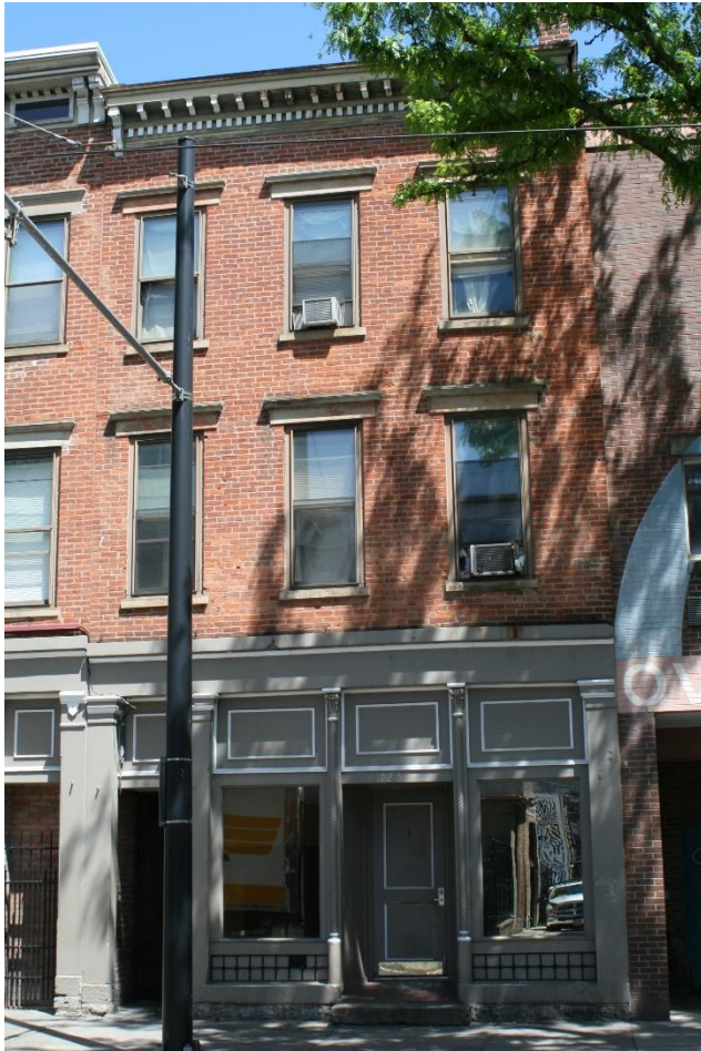
West Façade – South End
