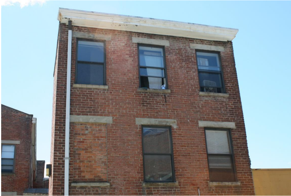
East Façade – Upper Windows and Roof
