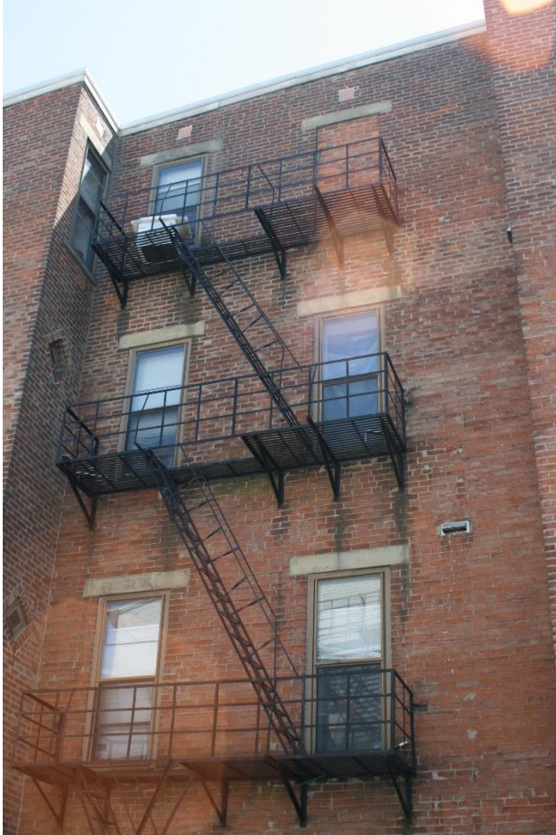
North Façade – Center Section
