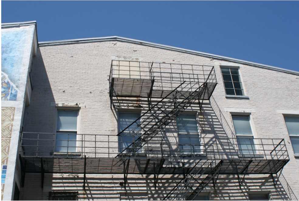
South Façade – East Side
