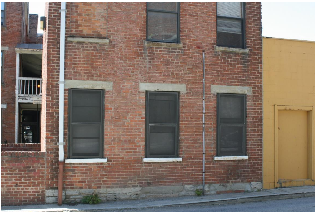
East Façade – Lower Windows and Roof
