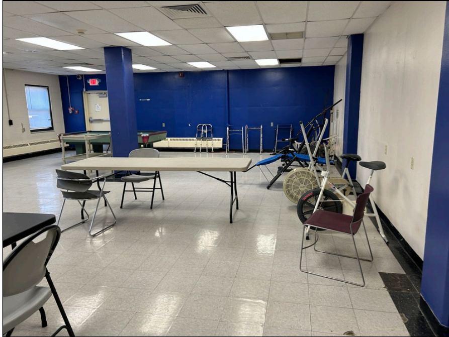
15 - View of typical finishes located within the Rec Room. View of HA-5 (Black Floor Tile w/ ACM Black Mastic), HA-6 (White Floor Tile w/ ACM Black Mastic), and HA-10 (2'x4' Pin & Fissure Ceiling Tile)
