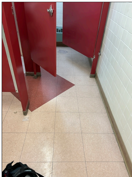
16 - View of HA-11 (12"x12" Red Floor Tile w/ ACM Black Mastic), HA-12 (12"x12" Light Pink Floor Tile w/ Yellow Mastic), and HA-19 (Cream Cove Base)
