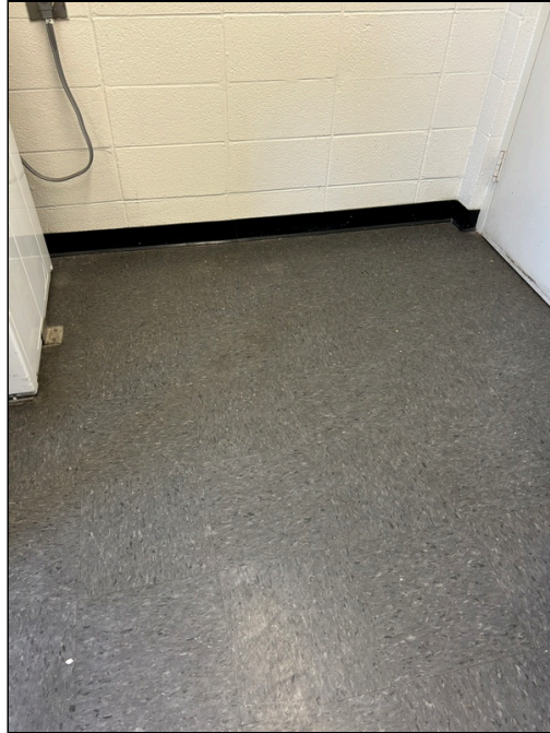
19 - View of general finishes located in the Laundry Rooms. View of HA-16, 12"x12" Dark Gray Floor Tile w/ Yellow Mastic.
